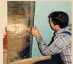
Positioning the board and fastening with screws
